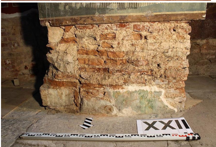
Fig. 9.: South-West semi- pillar. Vertical seam in the center of the pillar. View from the North
