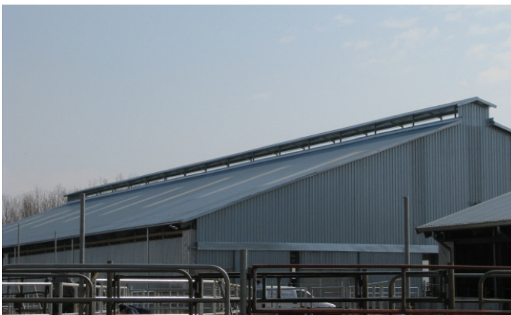
Photograph 1: Freestall dairy barn with natural ventilation, Jászapáti
