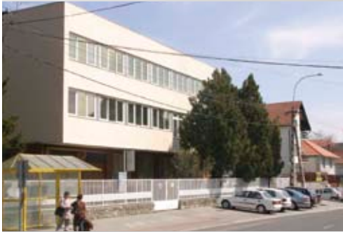
FURTHER TRAINING AND CONFERENCE CENTRE OF THE PRISON SERVICE (PILISZENTKERESZT/IGAL)
