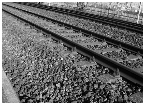
1. ábra. Vasúti pálya zúzottkő ágyazata Aggregates in the construction of railway track
