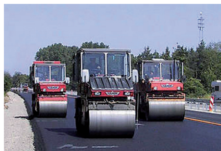
"Porous asphalt" designed for noise reduction
