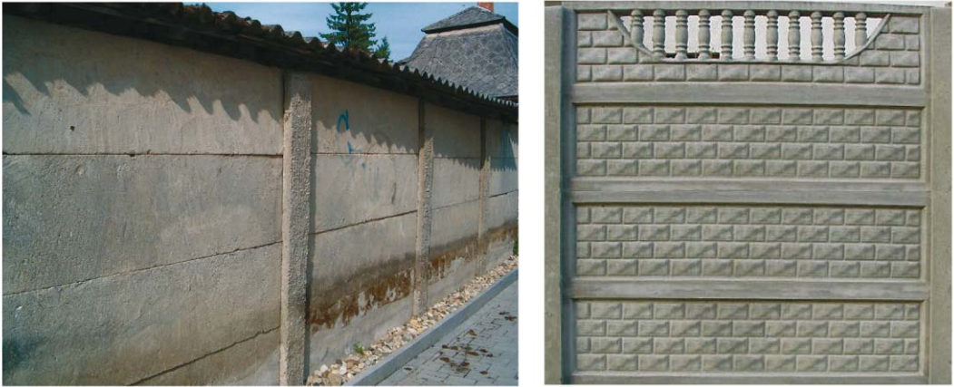
Figure 1. Concrete fences: past and present [1]
