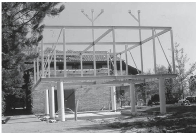
Figure 12. Picture of the structure during construction.
