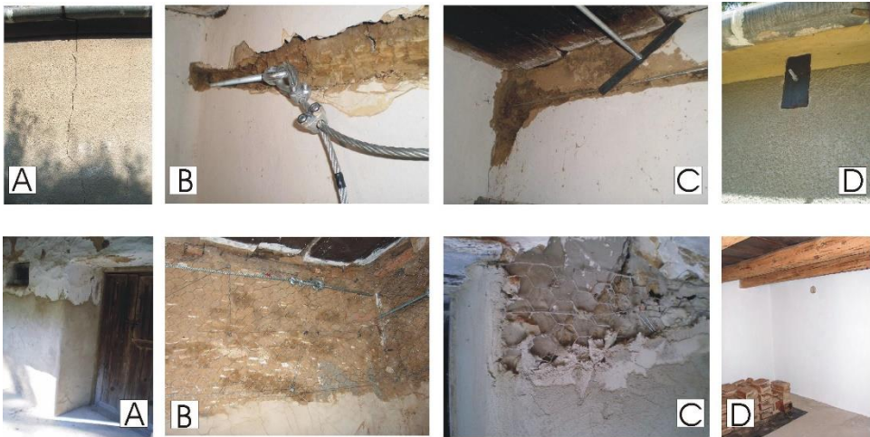
Figure 8, 9. Two renovation processes of the adobe house. Upper part: strengthening of the of the walling: (A) splitting (B) connection of the cable-rope to the screw (C) The stretched cable-rope in inside (D) The screw with underlay in outside. Lower part: Strengthening of the surfaca: (A) the moulding surface in outside (B) the wire mesh mounted on the wall (C) rough-casting (D) polished plastering in inside. (Source: Experimental work by the author Á.N.)
