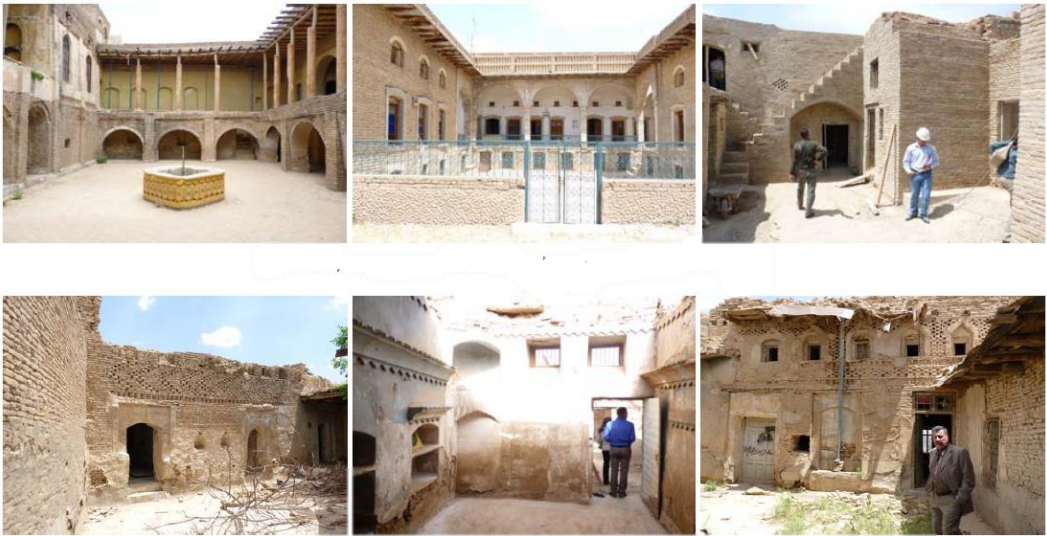
Figure 3: Erbil Citadel Houses renovations work. Reference: [4]
