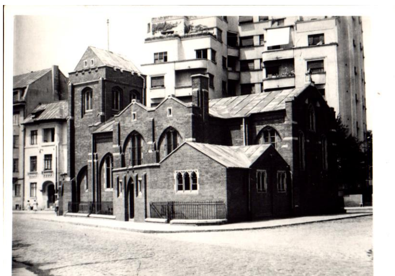
Figure 2 Photograph extracted from the Anglican Church's historical monument file - National Heritage Institute's Archives – File: FEV-B-II-M-A-19833. The southern and eastern elevations.
