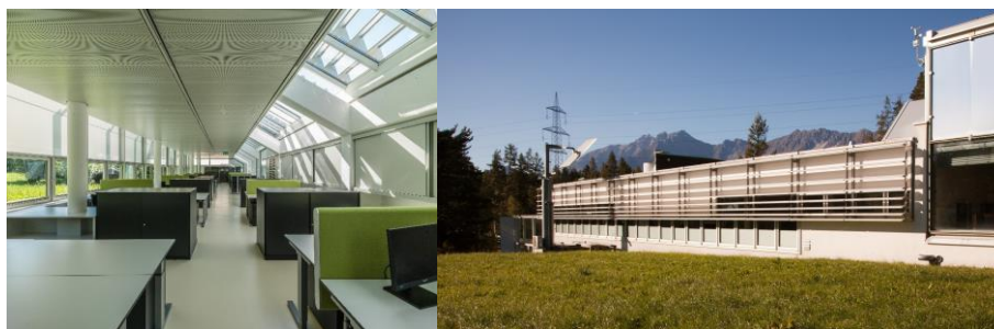
Figure 1 Interior (left) and exterior view (right) of the Bartenbach R&D building in Aldrans, Austria. In the right part of the interior area, the skylights of the north façade can be seen, the exterior view shows the static daylight system on the south façade.
