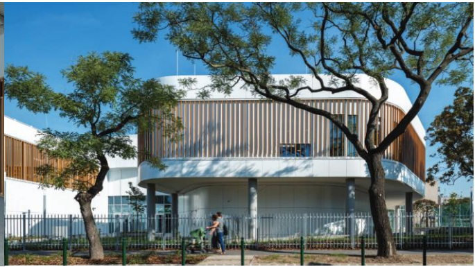
Figure 6. South wing of the Jedlik High School [12].
