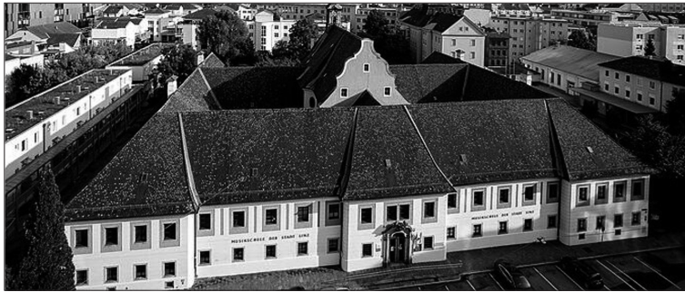
Figure 5. The building of the former Prunerstift in Linz, partially used as madhouse between 1788 and 1867. Recent view, photography taken by Volker Weihbold, Oberösterreichische Nachrichten (by courtesy).
