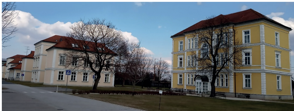
Figure 9: The former barracks on Kassai Road Source: Photo by János Perge.
