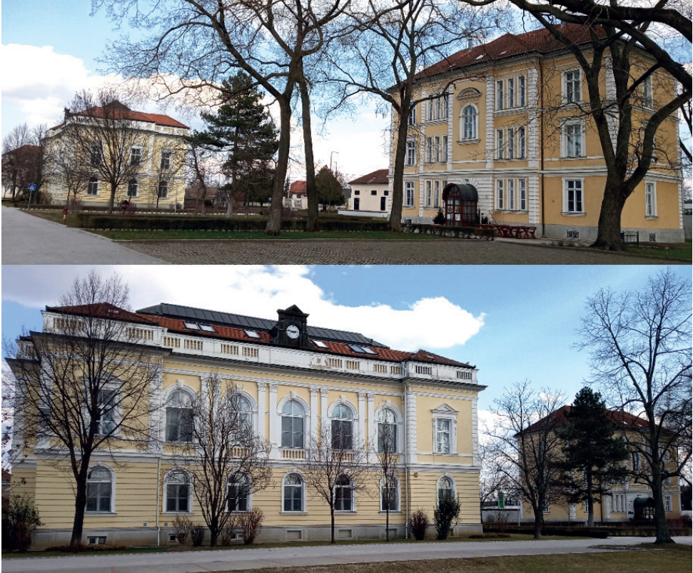
Figure 1: The former barracks on Kassai Road Source: Photo by János Perge.
