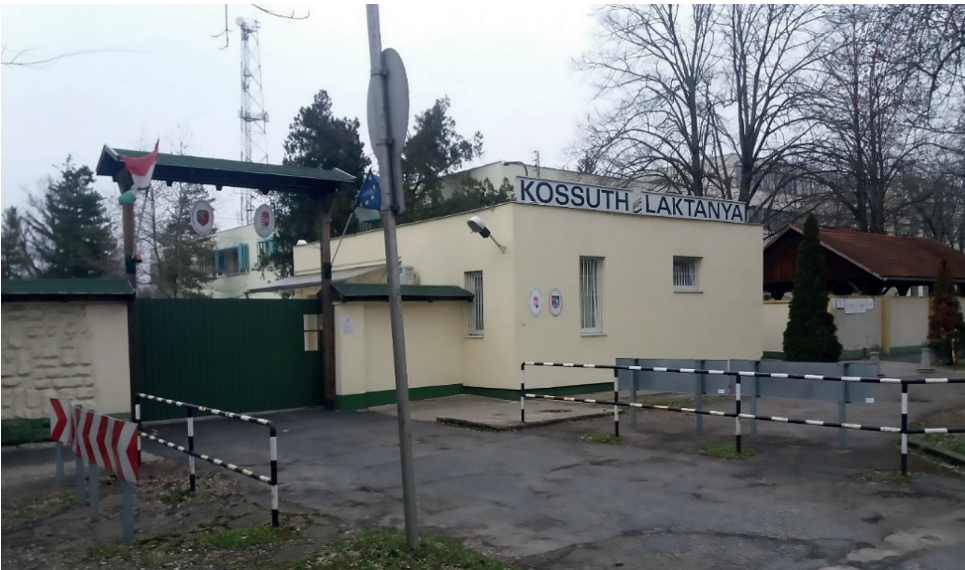
Figure 14: Kossuth Barracks Source: Photo by János Perge.
