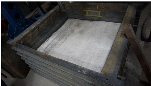
Figure 2. The high strength geotextilie on the sand layer
