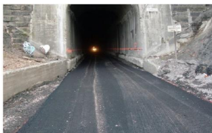
Figure 5. Asphalt layer under ballast [3]
