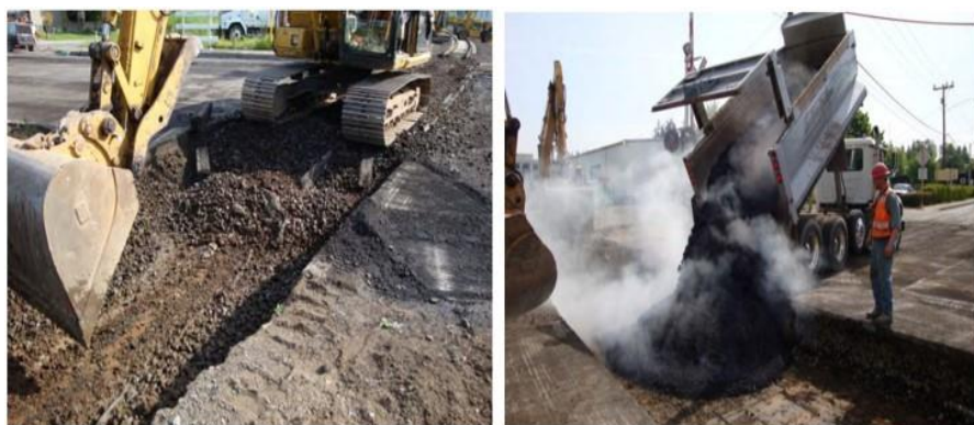
Figure 10. Rail/highway crossing rehabilitation. [1].
