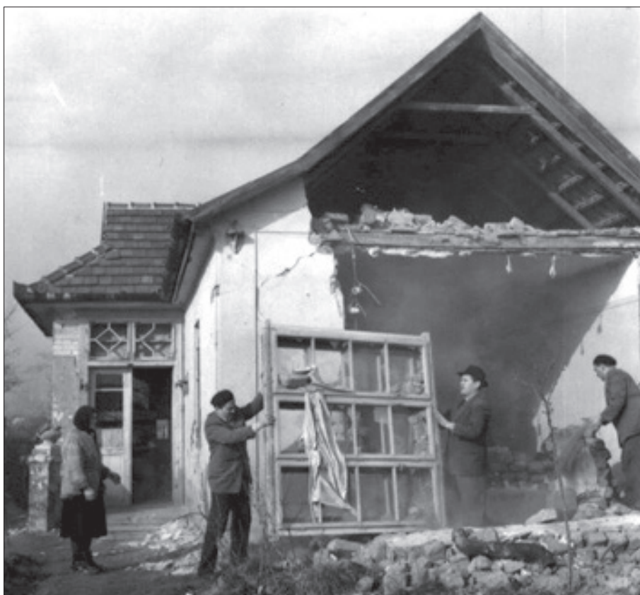
Photo 1. Earthquake aftermath in Dunaharaszti in 1956 (M 5.6; I0 8). Some 3,144 buildings were damaged out of the 3,500 in the epicentral area. Fall of gable walls as shown in the picture were typical building damage in an area of about 37 km radius. Source: Geodetic and Geophysical Research Institute of HAS
