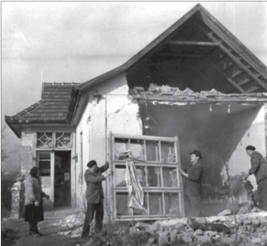
Photo 1. Earthquake aftermath in Dunaharaszti in 1956 (M 5.6; I0 8). Some 3,144 buildings were damaged out of the 3,500 in the epicentral area. Fall of gable walls as shown in the picture were typical building damage in an area of about 37 km radius. Source: Geodetic and Geophysical Research Institute of HAS
