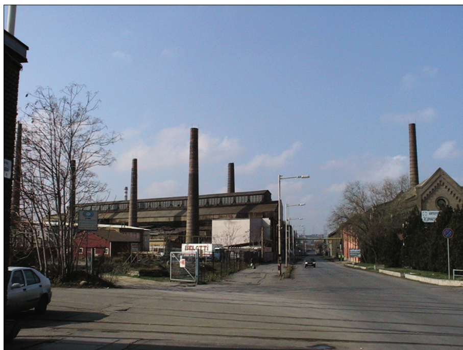
Photo 1. Part of the Csepel brownfield industrial park (Photo by Kiss, É.)
