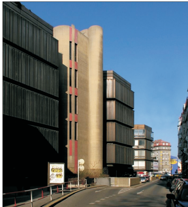
Photo 1. Massive concrete building of the Kotva shopping center. (Photo: SIKOS T, T.)
