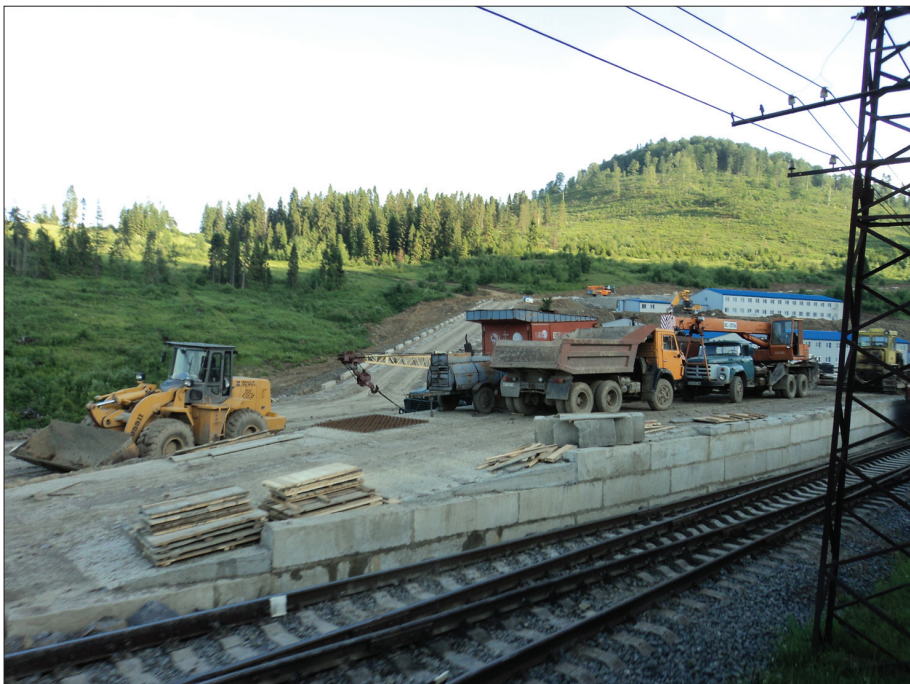
Photo 3. Construction of the new Beskydskyi tunnel
