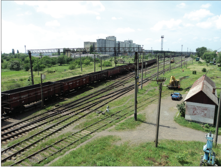
Photo 2. The modernised freight station of Uzhgorod II
