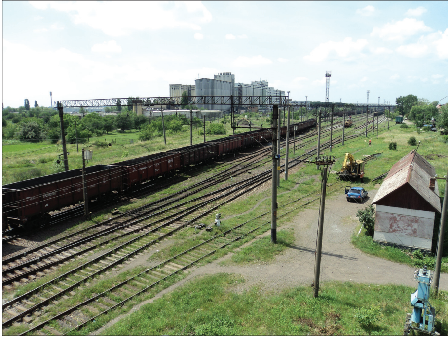
Photo 2. The modernised freight station of Uzhgorod II
