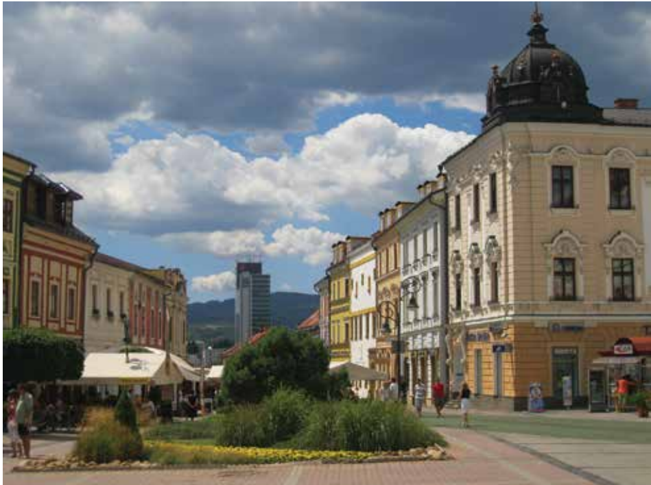
Photo 2. Entrance to Dolná ulica (Lower Street). Photo by Brrušíková, A. 2017.
