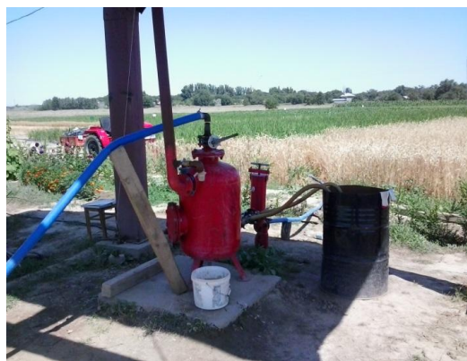
Figure 3. Water cleaning and additional fertilizing system
