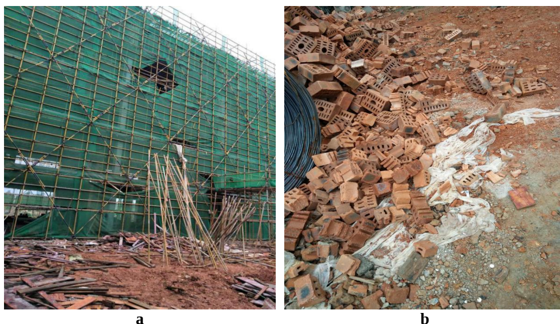
Figure 4. a. Waste wood. b. Discarded bricks
