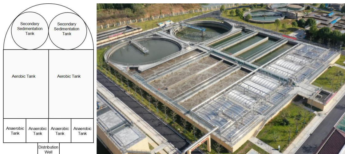
Figure 3. Phase II expansion of AAO biochemical combined pools
