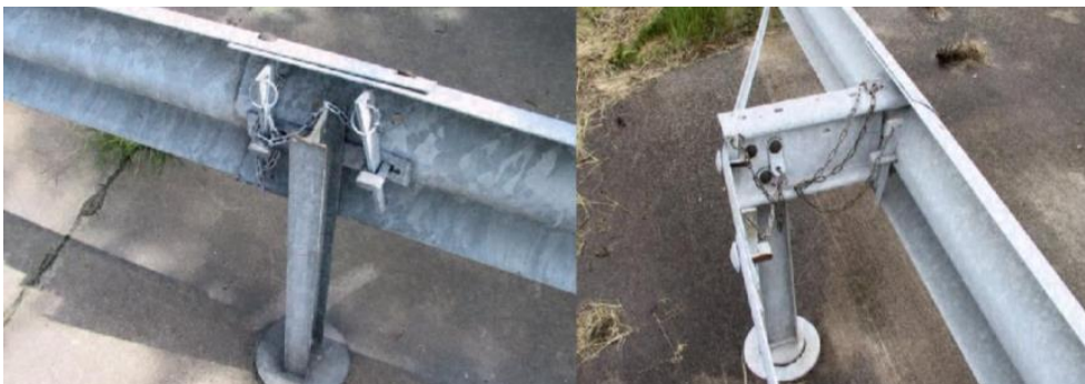
Figure 6. „Specially designed, quick-release tape barrier.” 21
