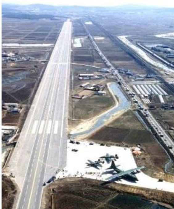
Figure 5. „Emergency landing site Suwon, South Korea” 18
