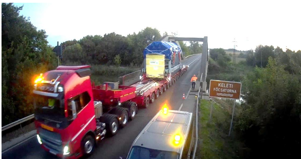
Figure 2: Civil overload transport on the bridge (photographed by the author)
