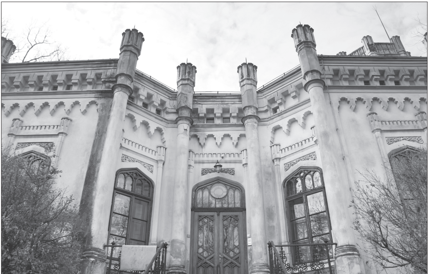
■ Foto 5. Accesul principal ■ Photo 5. Main access
