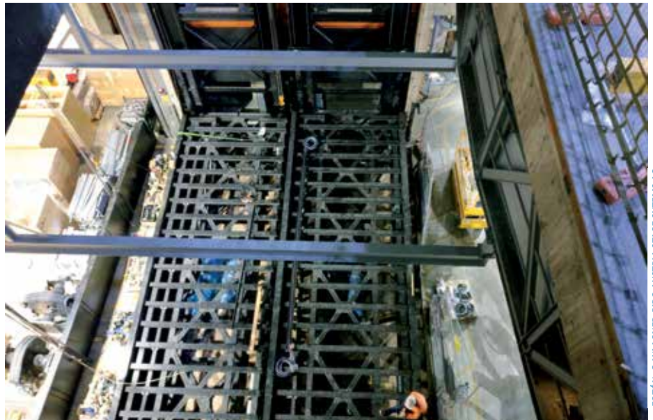
FOTÓK: © WAAGNER-BIRO AUSTRIA STAGE SYSTEMS AG
