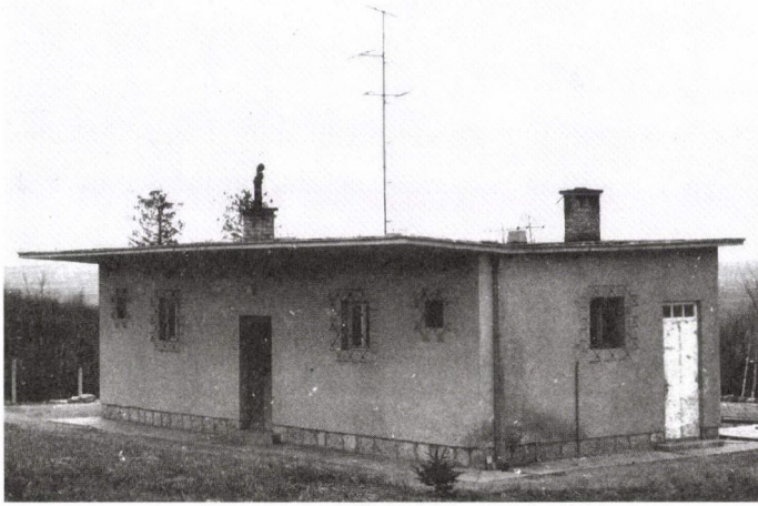
Fig. 2. The building in which the earth currents are recorded (bureau building)
