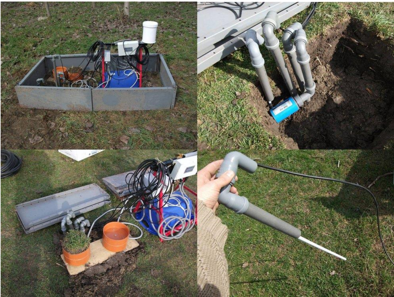
Fig. 2 Installation of the measurement stations
