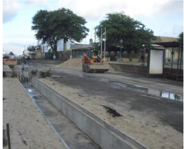
Fig. 9 Torrential correction works near Praça Estrela in December 2010
