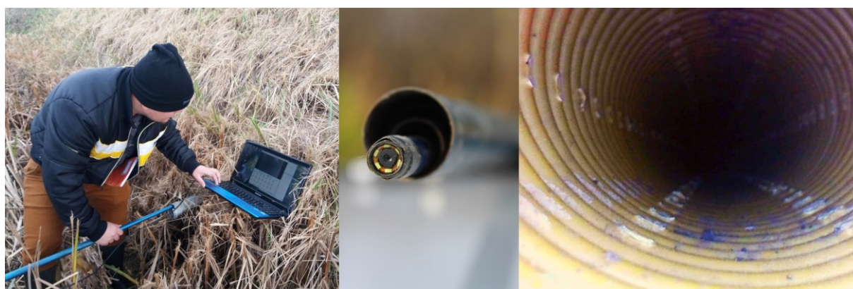
Fig. 9 The inspection of drain outlets and inner sections by endoscope camera
