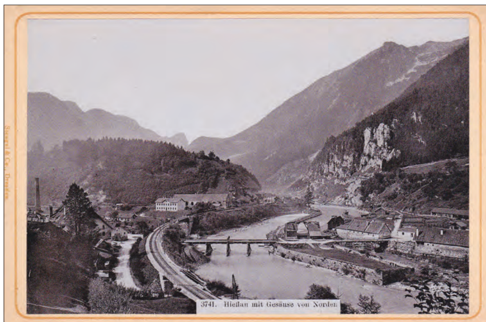
Figure 8 The Enns rake at Hieflau in 1896 (collection Reismann)
