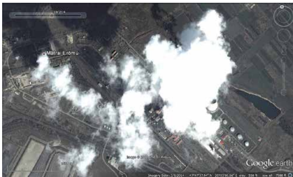
Fig.3. First type of plume merger in the Mátra Power Plant, Hungary.
