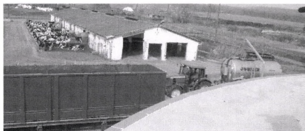
Figure 2. Biogas-plant built in the neighbor of dairy farm. (Source: own collection)
