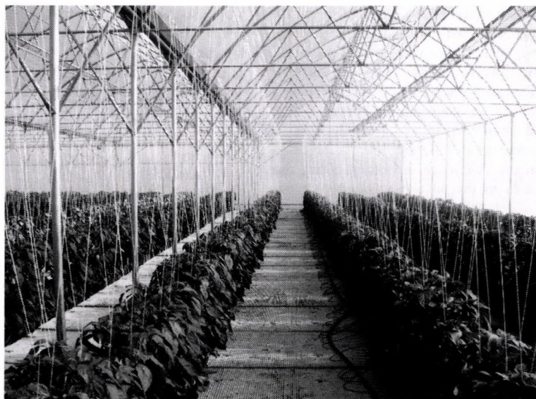
Figure 2. The Hydroponic growing in the experimental concrete panel heated 780 m 2 greenhouse.
