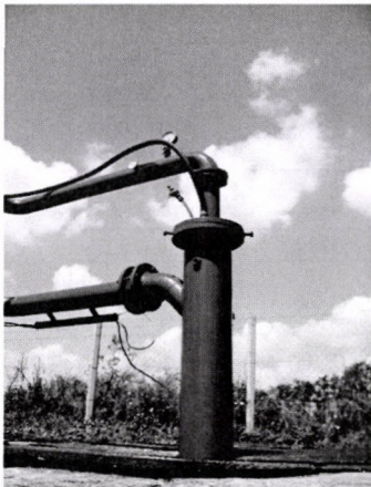
Figure 2. Thermal well with diving-pump excavation
