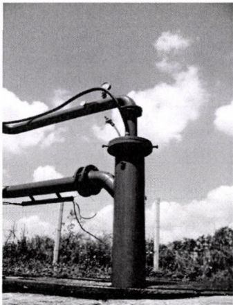
Figure 2. Thermal well with diving-pump excavation
