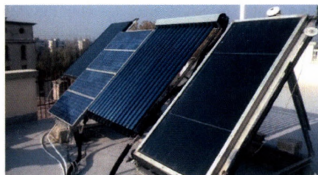
Figure 1. Solar collectors at the department, among them the vacuum tube collector (2 nd ), used or the experiments
