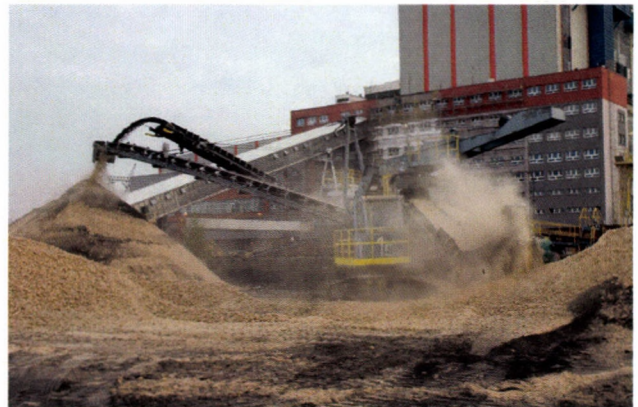
Figure 8. Production of the coal and biomass mixture for the cogeneration process
