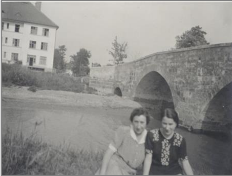
Picture 2: The old bridge that connected the two settlements 5
