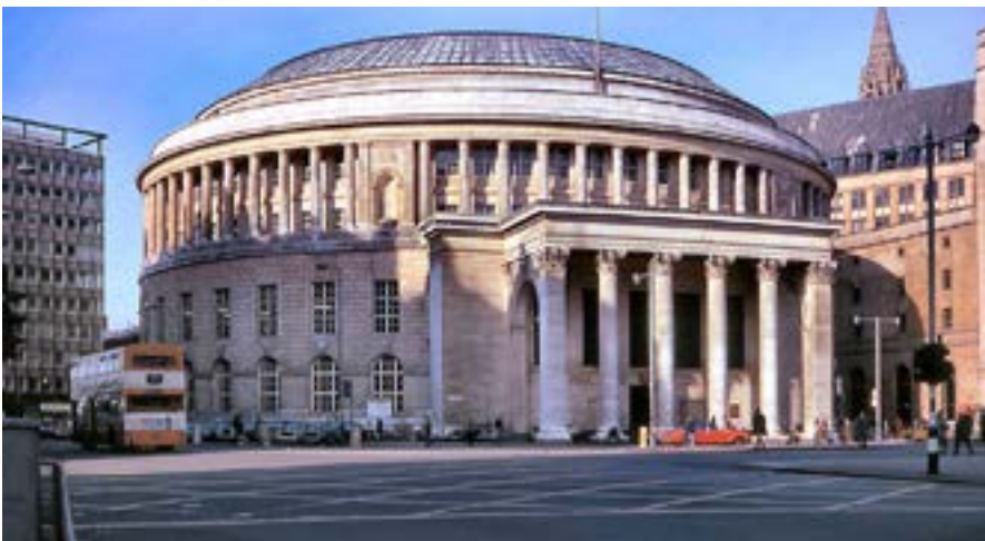
Figure 3. Manchester Central Library
