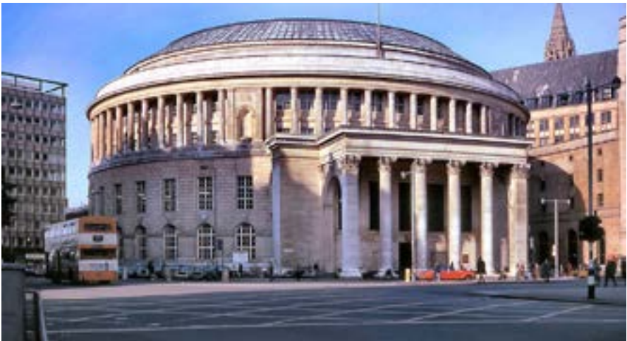
Figure 3. Manchester Central Library
