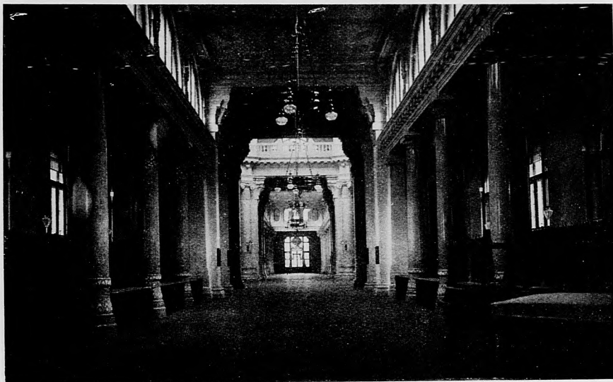
THE HALL OF THE NEW STOCK EXCHANGE.
