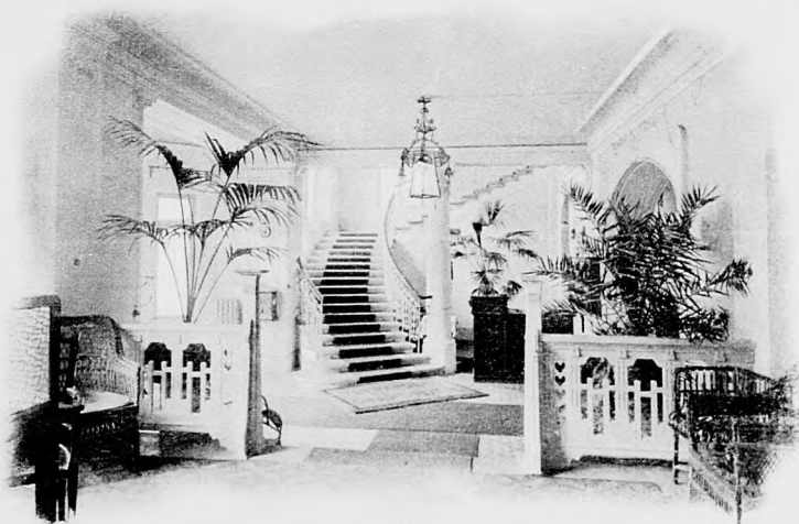
STAIRCASE OF THE GRAND HOTEL TÁTRA-FÜRED.
