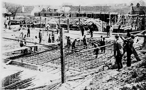
SHEWING THE IRON BETON FLOORING OF THE NEW BATHING ESTABLISHMENTS AT VIZAKNA.
