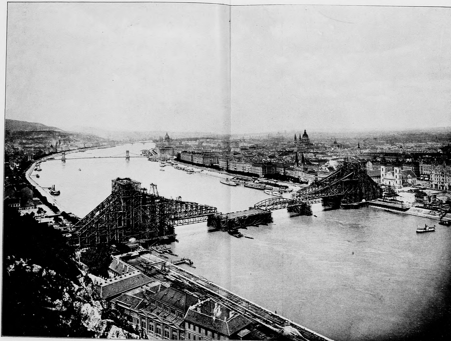
ELIZABETH BRIDGE: FURTHER PROGRESS; THE TEMPORARY COLLAPSIBLE BRIDGE REMOVED.
